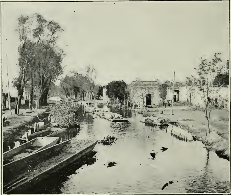
LA VIGA CANAL, FEDERAL DISTRICT, MEXICO.
